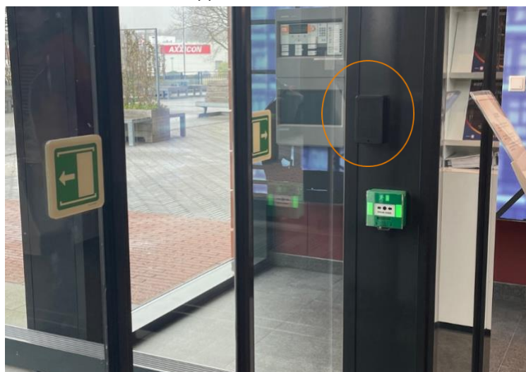
Figure 6: People counter at the central entrance on the ground floor (the emitter is circled orange).
